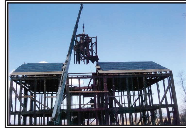
The process in pictures: Litchfield, when it was at the Industrial Park; disassembly; transport by flat bed truck; reassembly (note the spiral staircase being lowered through the roof), and the finished product in its new setting.
