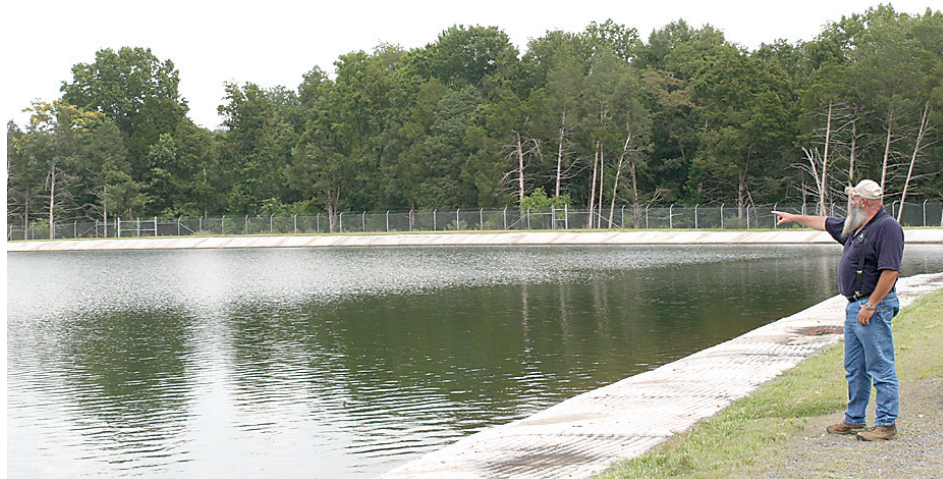
Dwight Baker says the five-acre 45 million-gallon emergency raw water storage reservoir can keep the towns of Orange and Gordonsville in water for a month.
