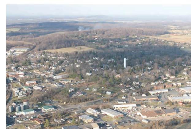
The photos above illustrate the complete water process for the town of Orange: from the intake at the Rapidan River, to Tim Hudson and Dwight Baker at the water treatment plant, to a beaker of raw water on the left and a beaker of purified water on the right and finally to the standpipe and the citizens of the town.
