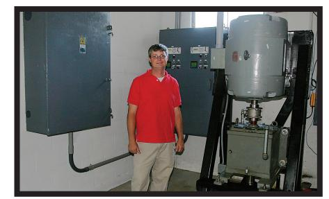
The heart of the operation. The water-powered rotating shaft comes out of the floor, through the square gear box and turns the keg-like generator on top. Electrical boxes behind Kevin O'Brien are crammed with high tech safety and remote control computer systems.
