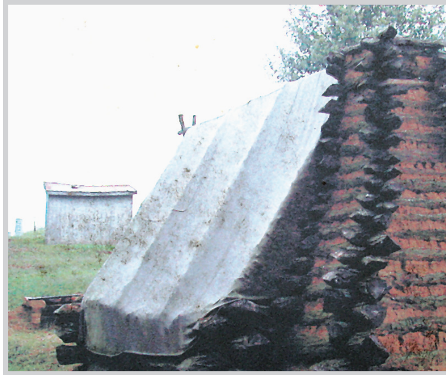
PHOTO BY PHIL AUDIBERT Re-enactors have reconstructed a typical winter quarters shelter at Montpelier. Earth chinking filled the gaps between logs, and a tarp over a ridge pole served as a roof. The hearth and chimney were made of earth and logs as well. A typical shelter is pictured at left.
