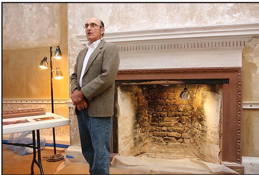
Photo by Phil Audibert Master mason and stone carver, Ray Cannetti hand carved the fireplace surround in the Madison drawing room from sandstone quarried in England.
