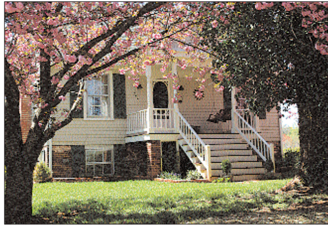
The 1850's toll keeper's house on the Blue Ridge Turnpike (Rt. 231) just outside Gordonsville.
