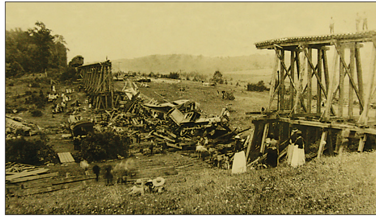
The wreck at the Fat Nancy Trestle, July 12, 1888.
