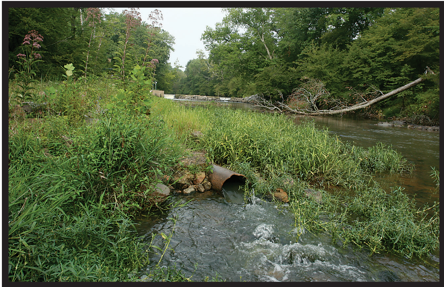
At a rate of about 700,000 gallons per day, treated effluent returns to the river from which it came. Note the spillway in the background where the intake for the town's water supply is located upstream.
